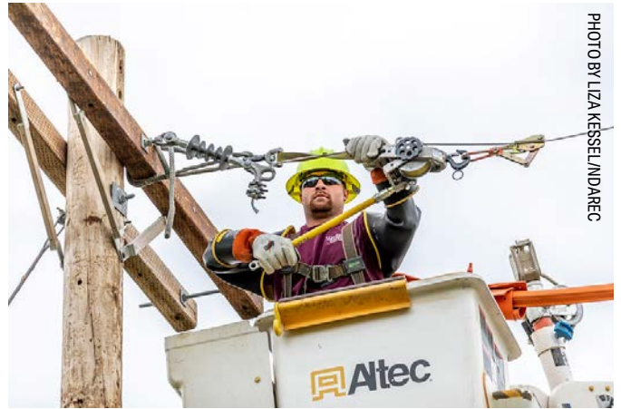
Laine Hoyt , Northern Plains Electric Cooperative lineworker, works on an energized line at Hotline School hosted by NDAREC.
